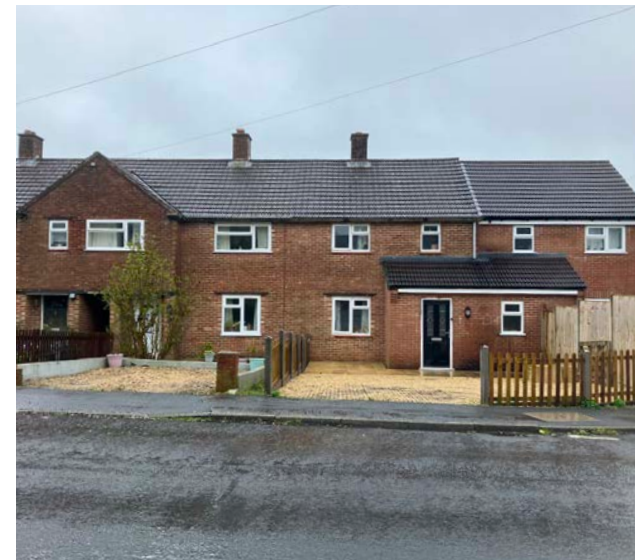
Figure 48: Red brick facade and concrete roof tiles, Lang Road.
