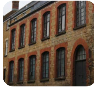
Archway access and window proportions.
