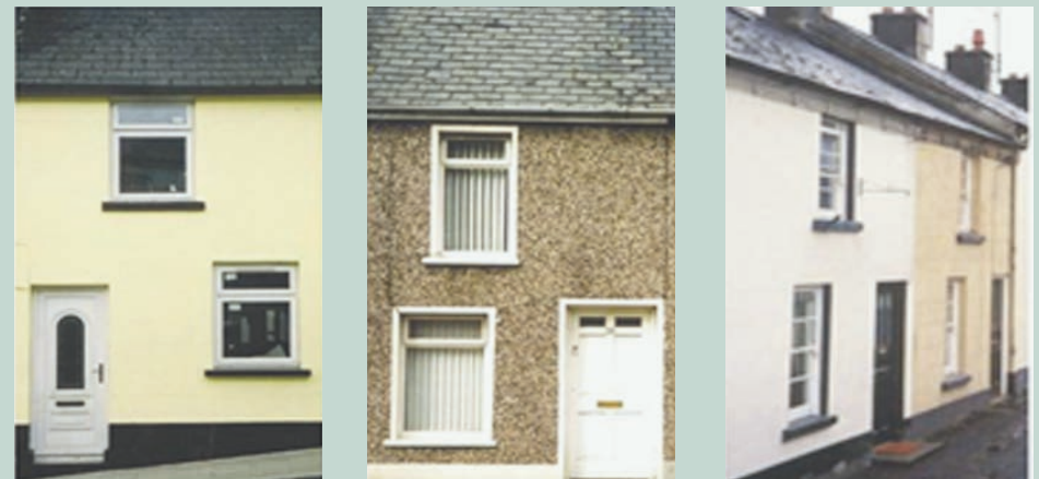
Figure 58: Example of original dwellings.
