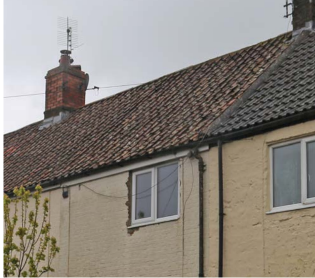
Figure 10: Single Roman roof tiles and dividing party wall upstand.
