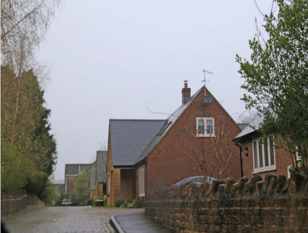
Figure 36: Private small development cul-de-sac. Higher quality external materials
