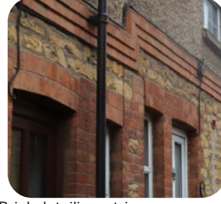
Brick detailing, string course and reveals.
