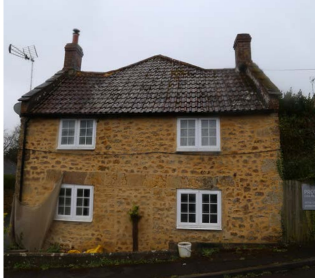
Figure 38: Traditional lime repointing/repair, clay double Roman tiles.
