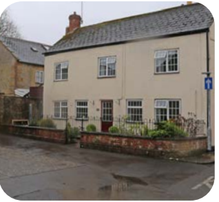
Enclosed garden frontages. Wall and railings.
