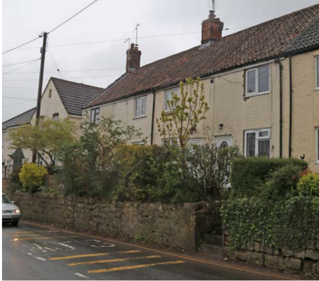
Figure 06: Properties elevated above busy access.
