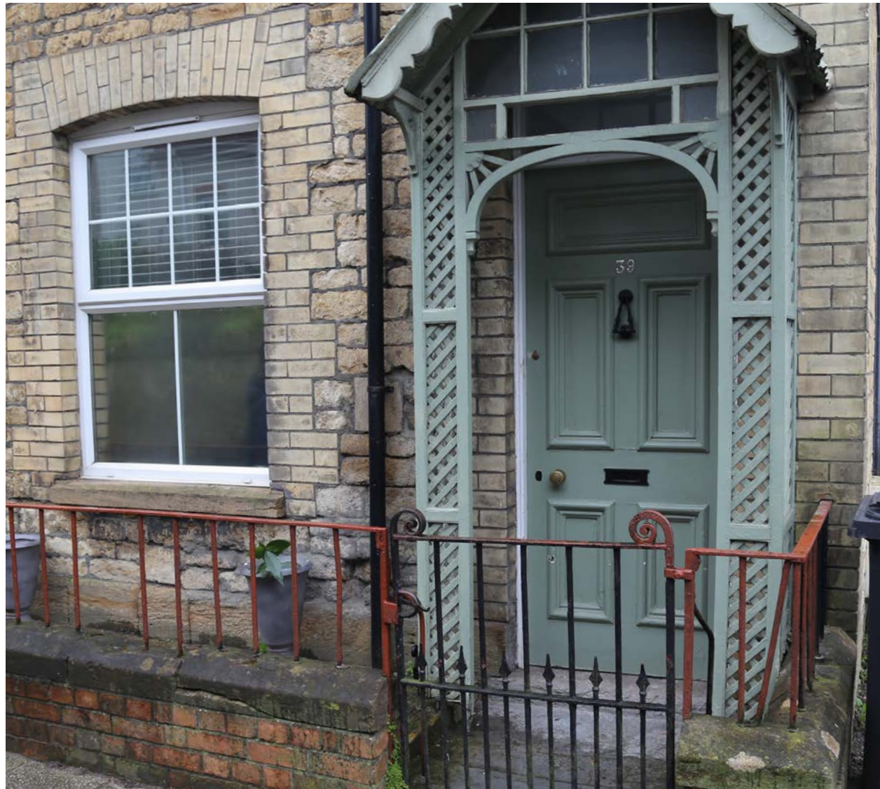
Figure 05: Layers of detail. Red brick garden wall, cut stone coping and railings. House plinth stone course, irregular sized stone used on façade, and buff brick reveals. Ornate semi-enclosed timber porch.
