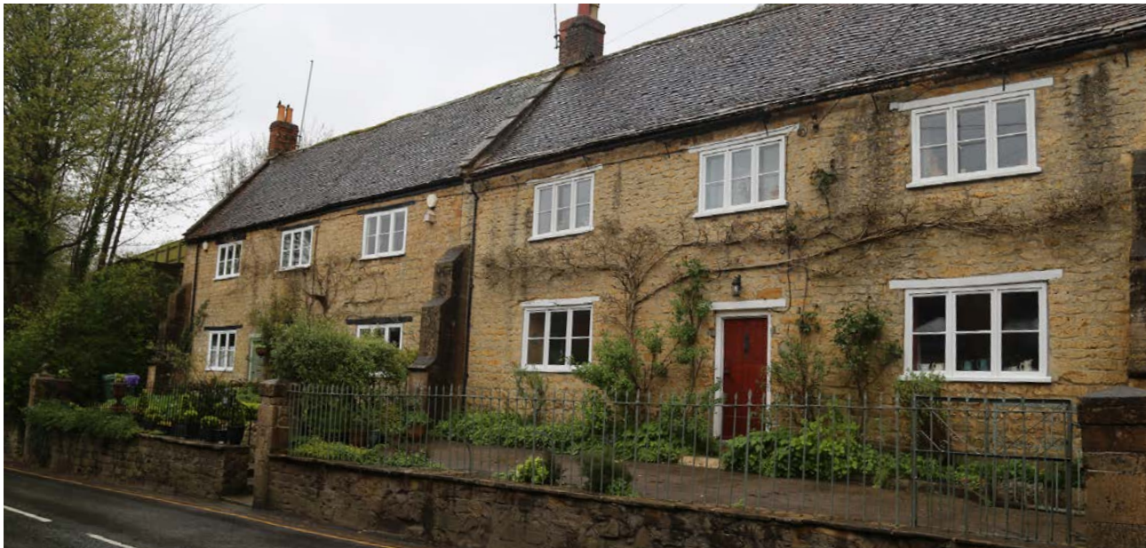
Figure 31: Stone buttresses, roof upstands and raised frontage.
