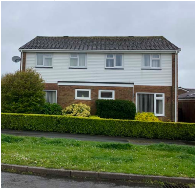
Figure 44: Semi-detached property with brick ground floor, white uPVC cladding on the first floor, and concrete roof tiles.
