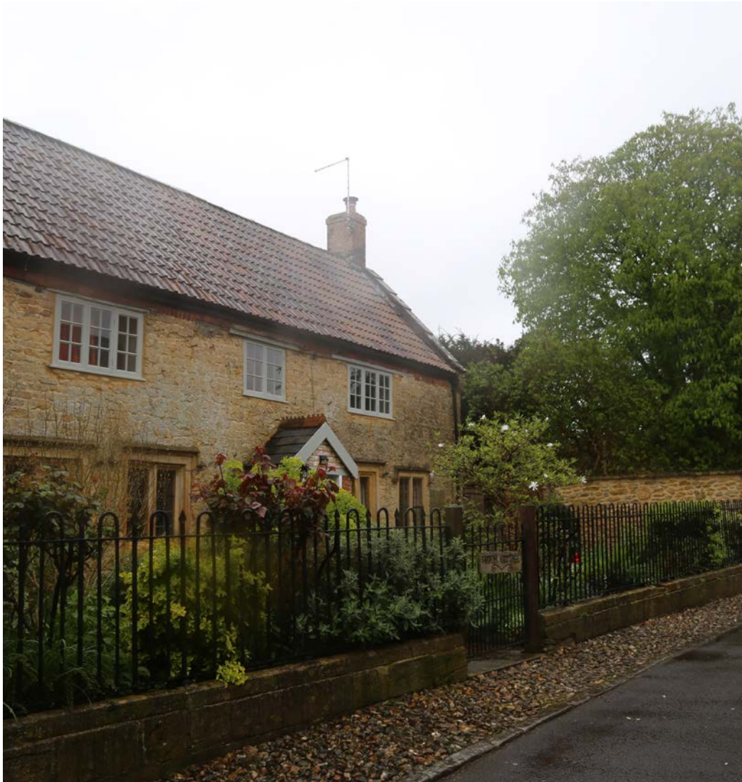
Figure 54: Red double Roman tiles, gable/verge upstands, upper three section casement (window).
