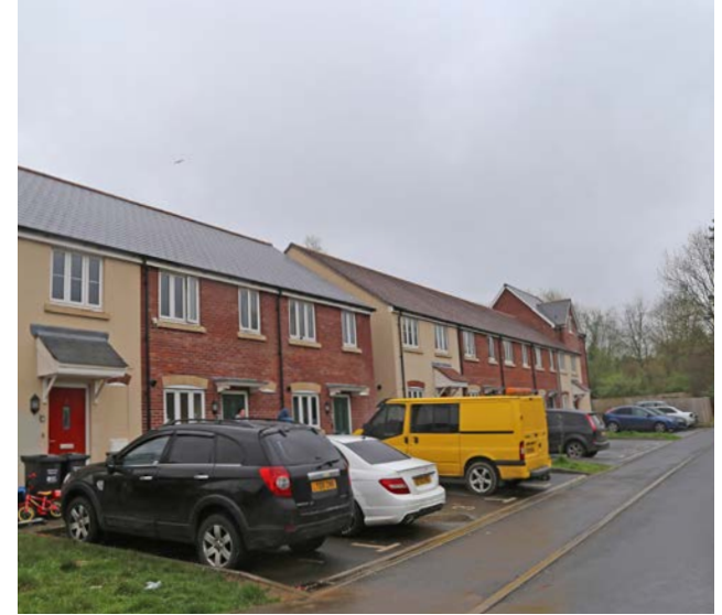
Figure 30: Recent development terraces fronting parking area.
