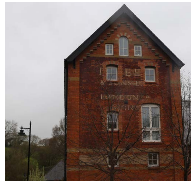
Figure 32: Brick constructed brewery.
