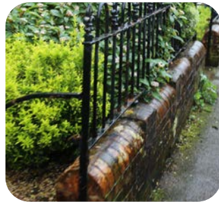
Brick dwarf walls with railings.
