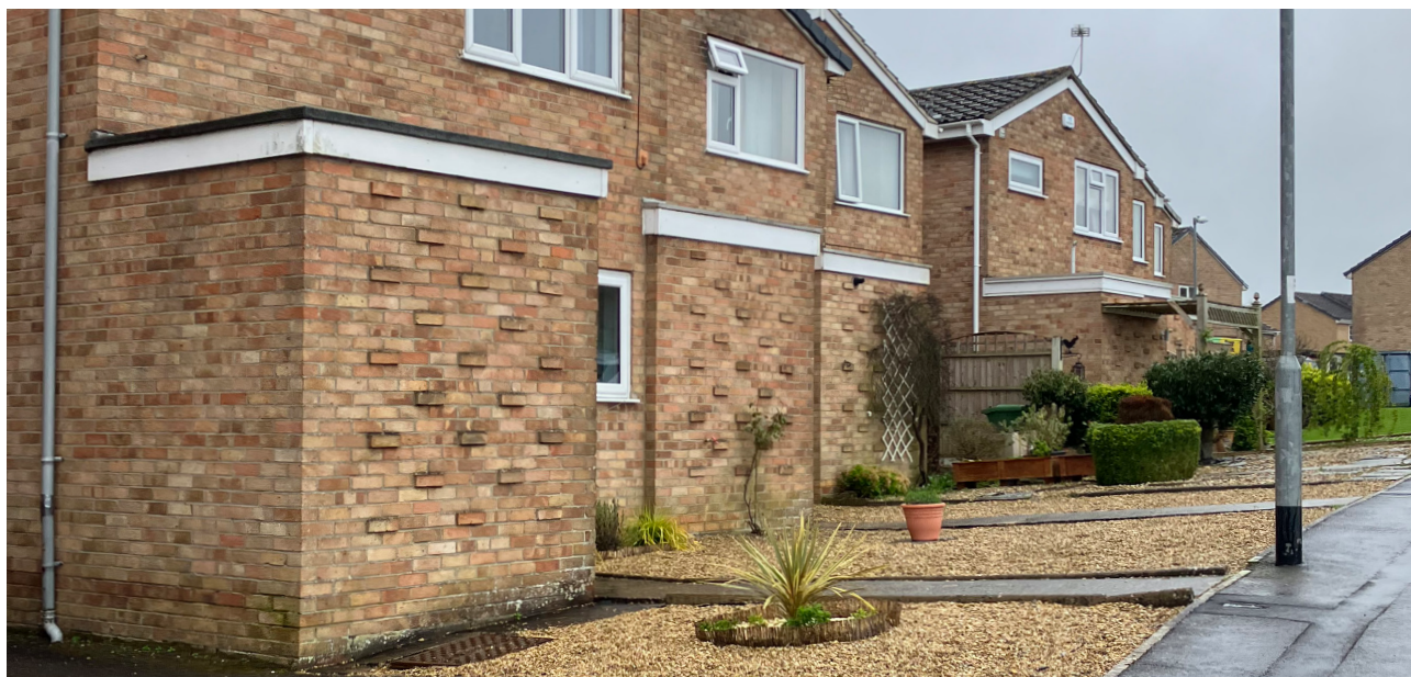
Figure 49: Simple brick detail appears in building and boundary walls.
